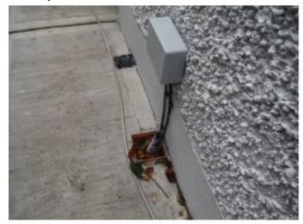
Lid required to cover where pipe exits the riser. to stop leaves and other rubbish collecting in the opening.
