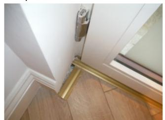
Flooring to be finished into corner at external utility door. Hinges need cleaning of paint spills.
