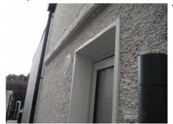
Vent for mechanical extraction in utility is installed but fan not installed. This is a requirement under current building regulations.
